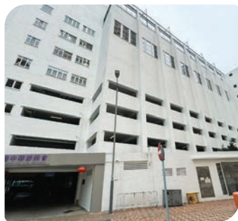
B座外牆 Renovation of external walls of Block B
