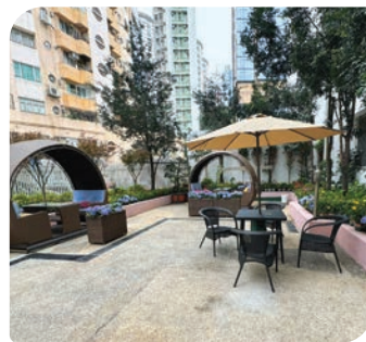
會員休息區翻新工程 Renovation of members' area
